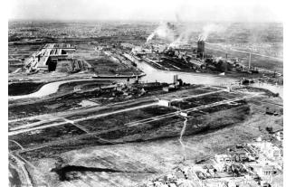
According to the Michigan State University Library, production began at the site on January 4, 1918, but according to Cabadas, the blast furnaces were still under construction in mid-January when Ford agreed to build 100 antisubmarine boats for the Navy.
